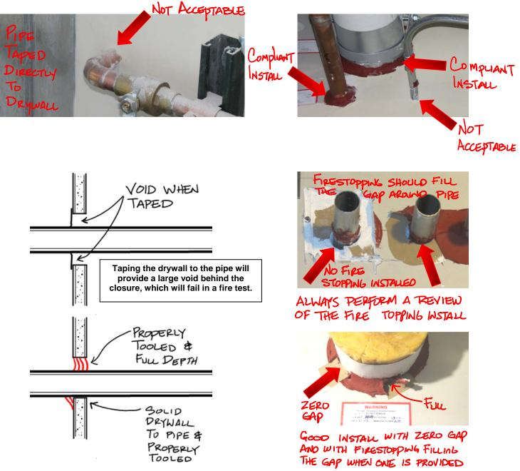
Obtain your UL Assemblies for each penetration from each trade as soon as possible, preferably, prior to the start of installation of the drywall so that your drywall contractor could build around the pipes to the UL Assembly the first time with tested design distance.
